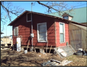
Before - Intern Kitchen
